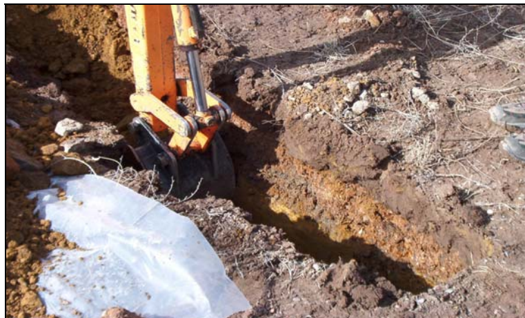
Photo 2. The trench shows the existing thin soil cover (i.e., cap) at Tailing Impoundment #3.
