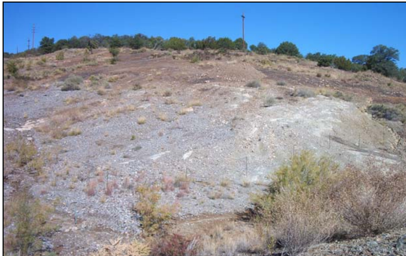
Photo 4. Barren eroding slope, north area.
