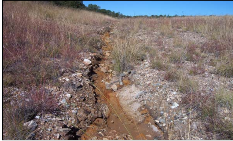
Photo 3. Run-off erosion demonstrating the need for improved drainages.
