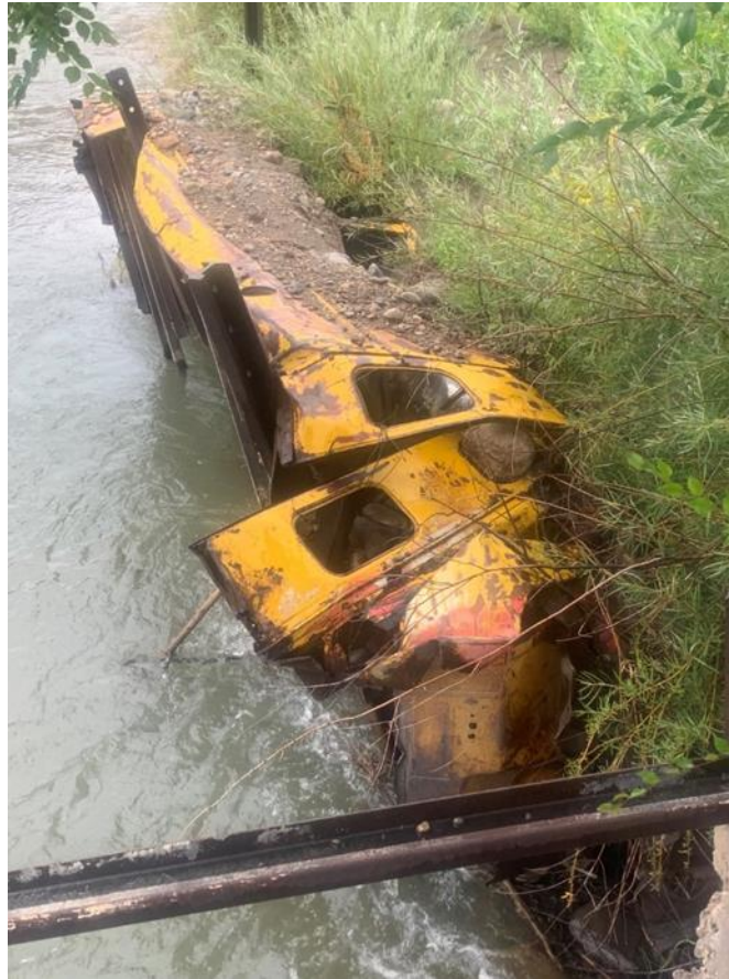
Figure 3.5. School Bus Placed at Cedar Ditch to Prevent Downstream Erosion
