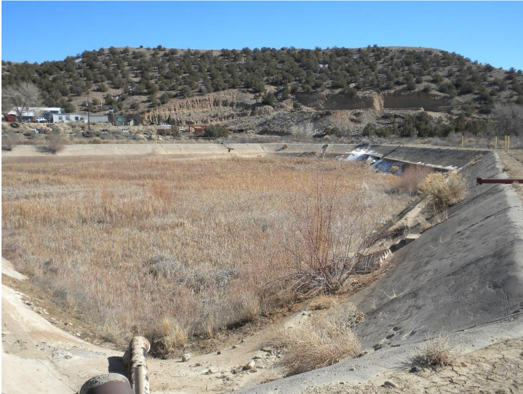
Figure 3.2. City of Aztec Water Reservoir 1. The reservoir is currently not in use, due to leakage issues. The vegetative growth visible in the photo has occurred during the period of disuse, will likely lead to further degradation of the structure.
