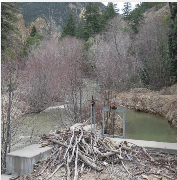
Current South Ditch Diversion structure.
